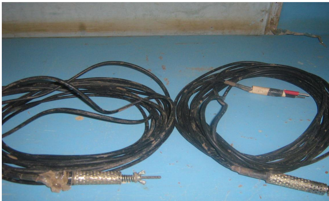
Figure 3: Reethorpes (moisture sensors).
