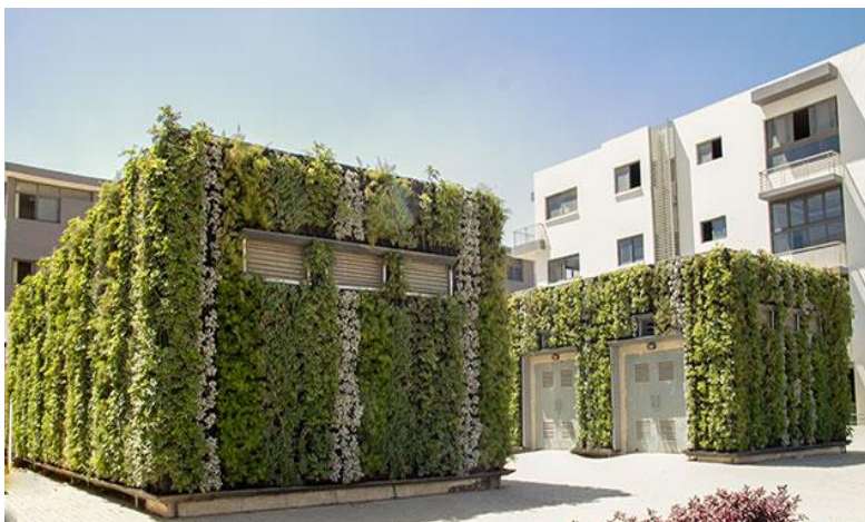
Figure 8: Living walls covering generator rooms with green walls in Taj City between Suez road and the ring road in Cairo ( https://schaduf.com/schaduf-projects/tag-sultan/ ).
