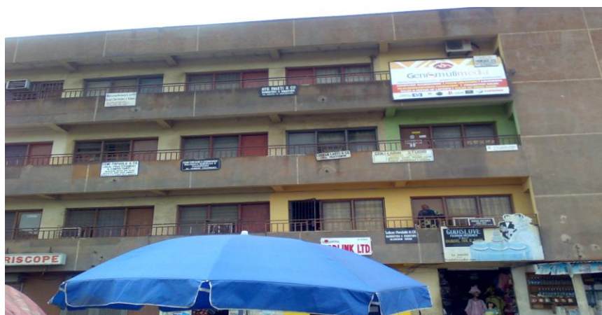
Figure 7. Three-storey building. Source: Field survey (2008).
