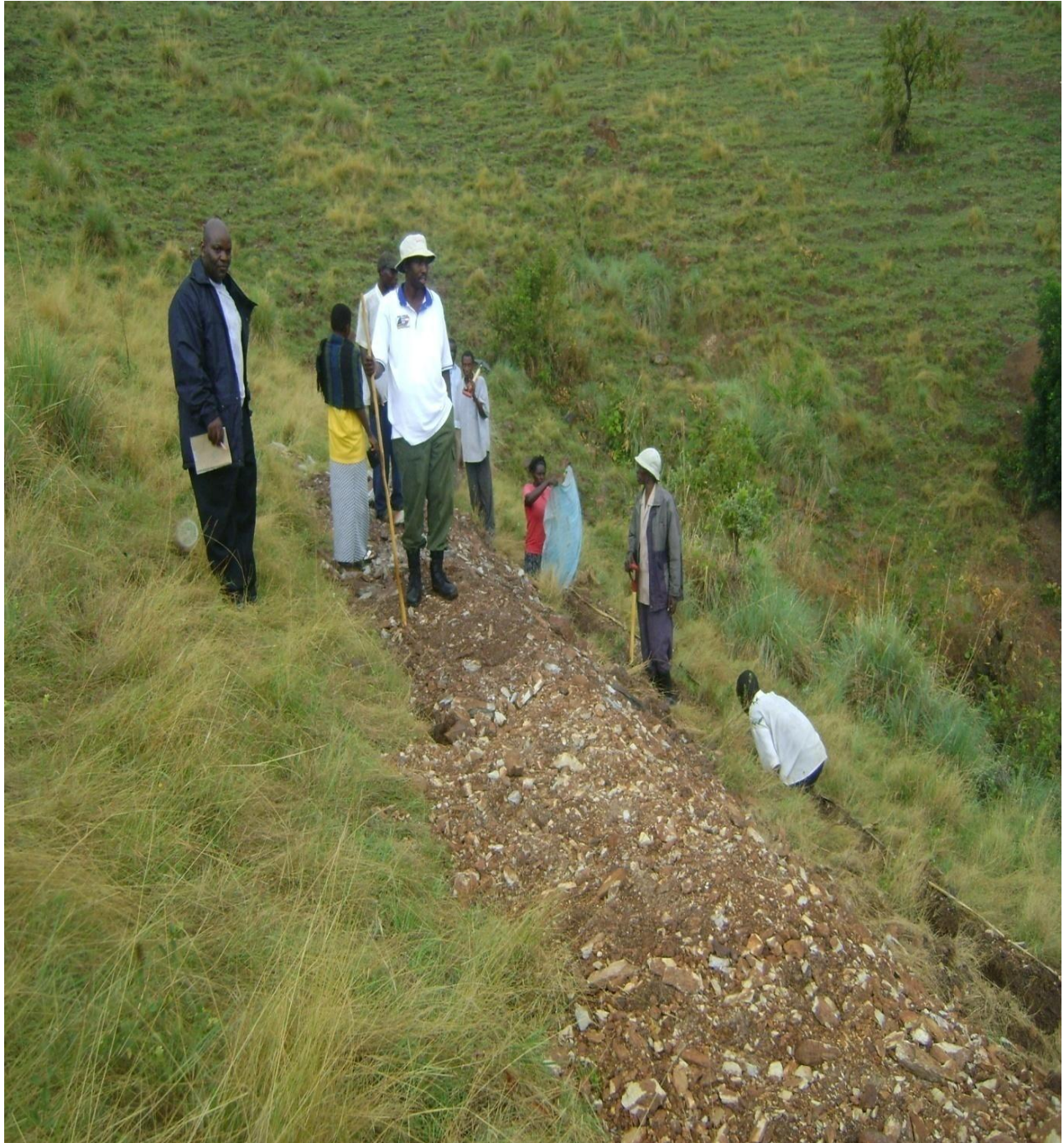
Figure 1. Digging of a trench on steep slope of Rwendama Hill in a white T-shirt and hat holding a stick is the District Natural Resource officer and in a black jacket holding a notebook is the author.
