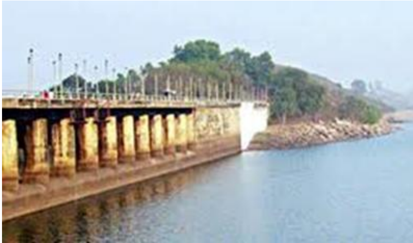
Figure 11. Tilaiya Dam upon the Barakar 15 .
