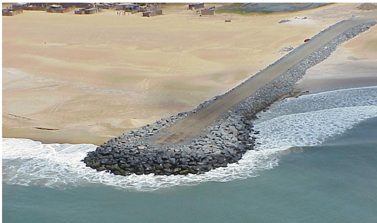
Figure 2. One of the six groynes along Keta shoreline (source: Google map).
